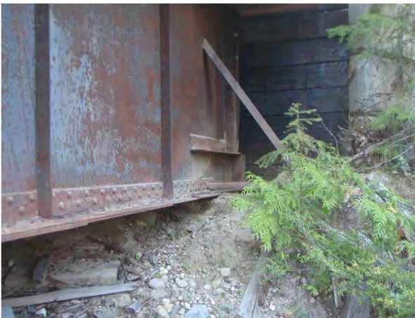
Figure 1-21: Camp end downstream bearing.
