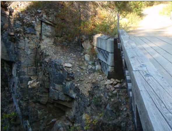
Figure 1-19: Camp end upstream wingwall.
