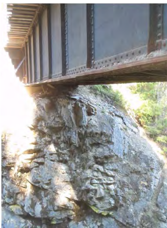
Figure 1-17: Camp end abutment.
