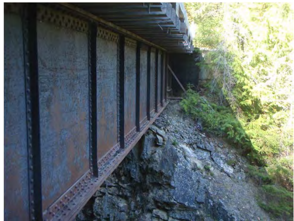
Figure 1-10: Downstream face looking towards camp end.
