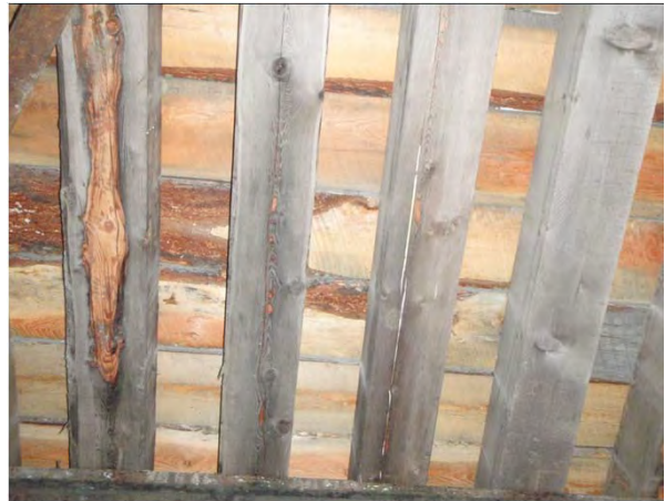
Figure 1-8: Underside of deck planks and deck ties.
