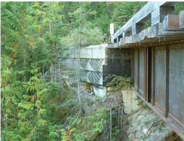
Figure 1-23: Woods end downstream wingwall.
