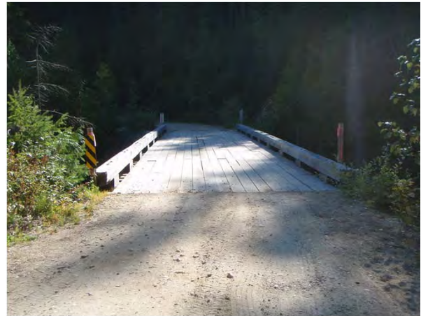
Figure 1-2: Looking towards woods end.
