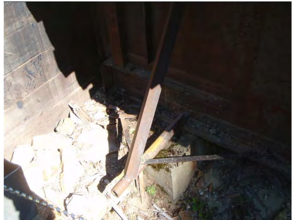
Figure 1-20: Camp end upstream bearing.
