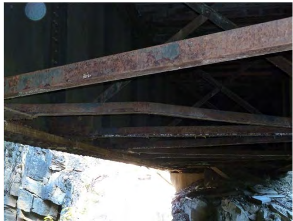
Figure 1-16: Bent plan brace near mid span.
