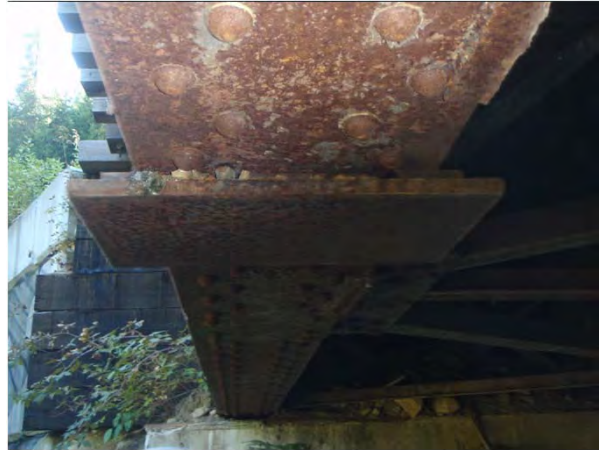
Figure 1-14: Plate welded to bottom flange of girders on woods end.
