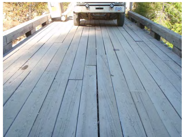
Figure 1-6: Typical running plank condition.
