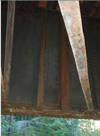
Figure 1-13: Additional stiffeners welded on interior face of girders.
