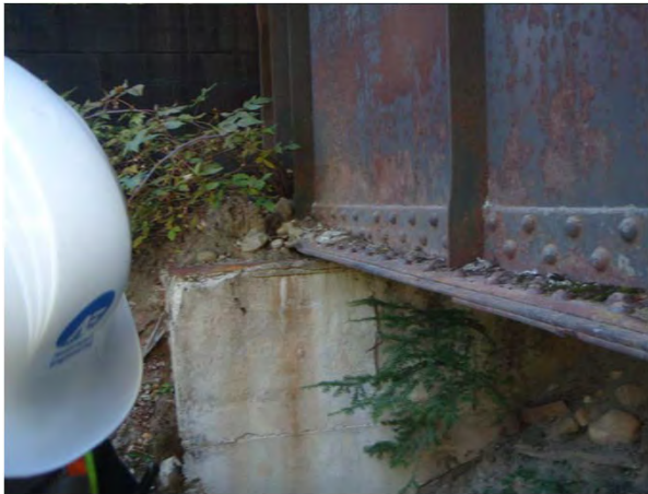
Figure 1-25: Woods end downstream bearing.
